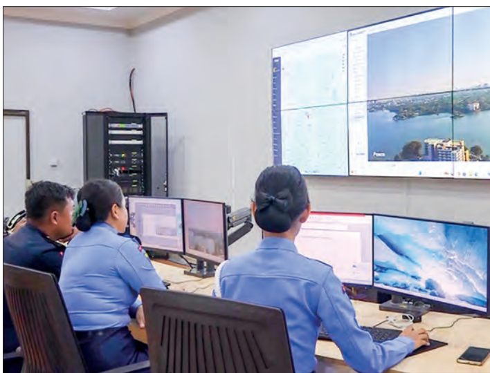
The Myanmar Fire Brigade Headquarters Command and Control Centre conducts the monitoring.
