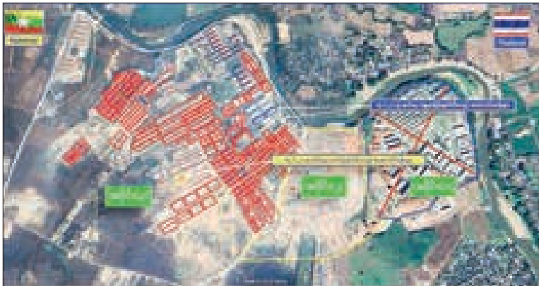
This map shows ongoing demolition measures in the KK Park Section 3.
