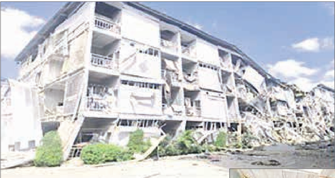
The completed demolition of a four-storey flat.
