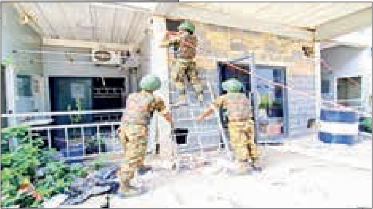
Security personnel are seen placing 151-kilogramme C12 to demolish the four-storey flat.
