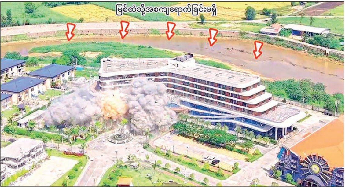
The systematic demolition of buildings and facilities in the KK Park area of Myawady Township, a hub linked to telecom fraud and online gambling.
