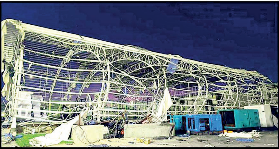
This photo captures the completed demolition of buildings and facilities in the KK Park area of Myawaddy Township.
