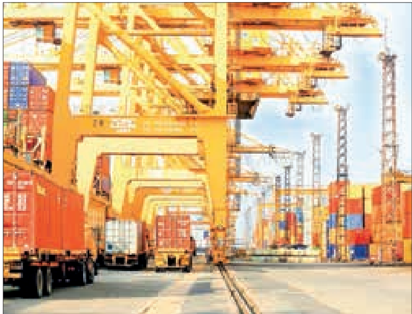
The ECT can now handle two ships at once along a completed 900-metre berth, with cargo moves supported by the project's latest automated systems. PHOTO: SRI LANKA PORTS AUTHORITY
