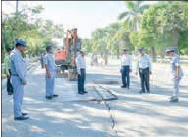
This photo shows the Nay Pyi Taw Mayor inspecting road repair work.
