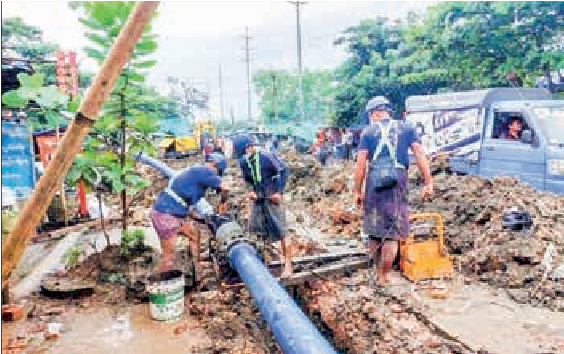
YCDC’s staff are seen connecting water pipes.
