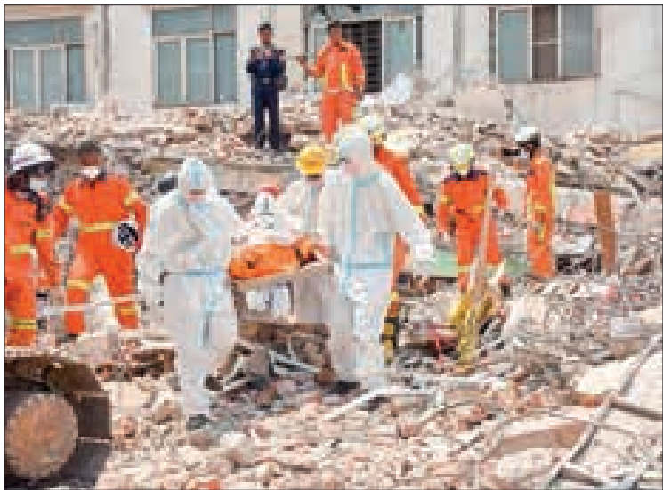
Bodies were recovered from collapsed buildings on 26 April.
