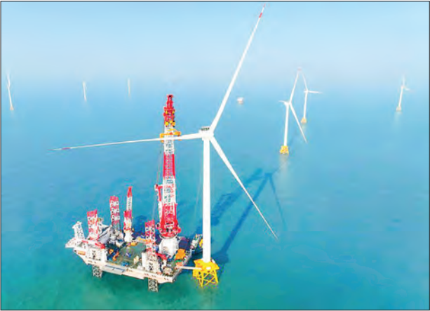
A drone photo taken on 13 January 2026 shows the construction site of a 20-megawatt offshore wind turbine unit in the coastal waters of southeast China’s Fujian Province. PHOTO: XINHUA
