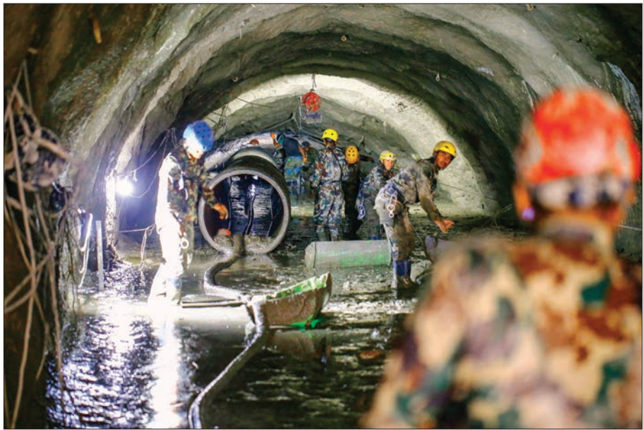
The Nepali Army conducts a search-and-rescue operation inside the Chilime Hydropower Station tunnel days after deadly flash floods and mudslides in Nepal's Rasuwa district on 10 September 2026. PHOTO: AFP
