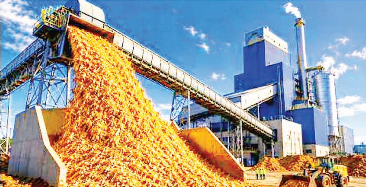
A biofuel power plant is seen in footage from an overseas news agency.
