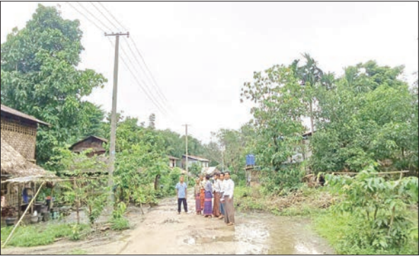
Officials inspect the completed power line installation in Kyauktaga Township.
