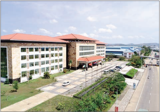
Aerial photo taken on 19 July 2022 shows the entrance of the Sihanoukville Special Economic Zone (SSEZ) in Preah Sihanouk province, Cambodia. PHOTO: SSEZ/HANDOUT VIA XINHUA
