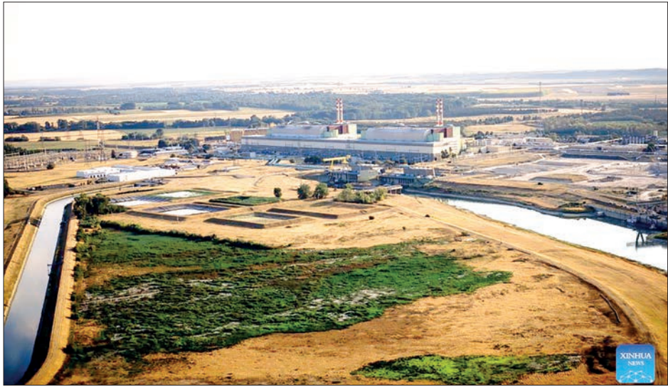
An aerial drone photo taken on 2 August 2026 shows a view of the Paks nuclear power plant near Dunaszentbenedek, Hungary. PHOTO: XINHUA
