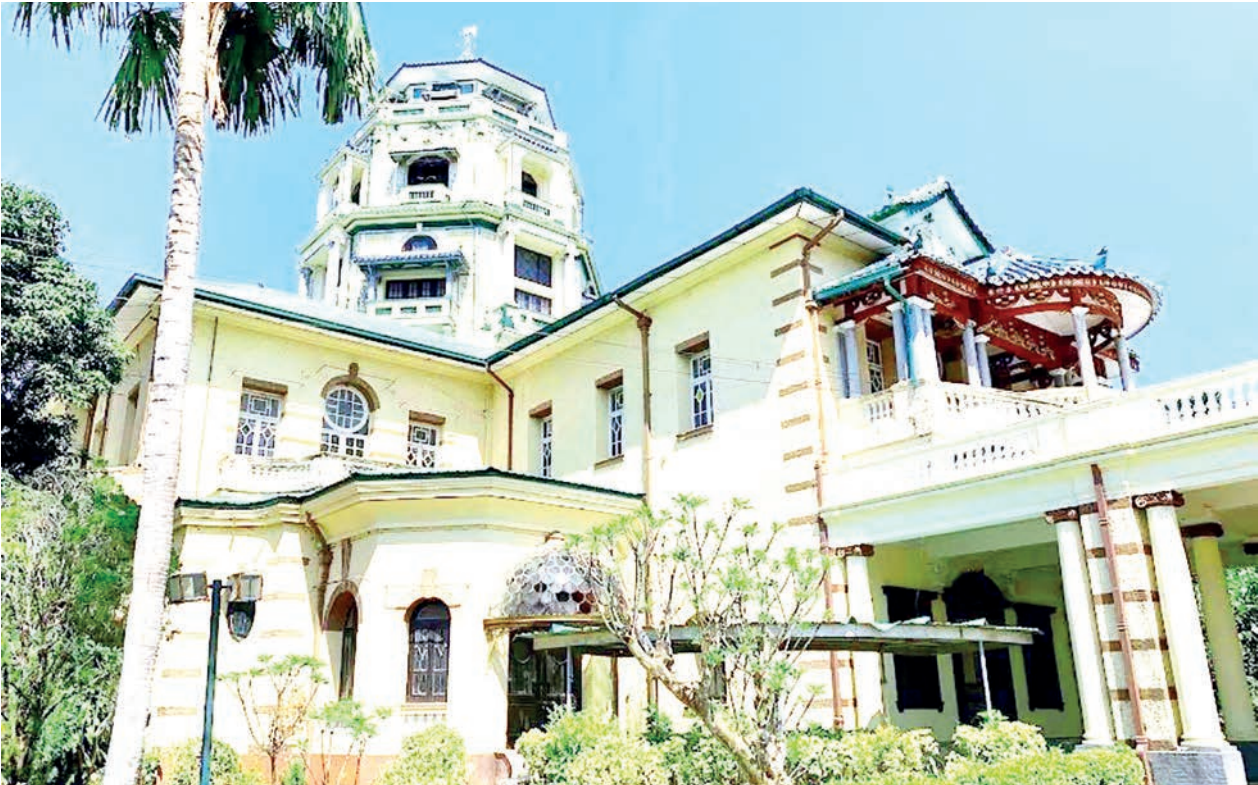
This image shows the Kanbawza Yeiktha (Chin Tsong Palace) in Yangon Region, where a bronze plaque marking its status as a heritage building is installed.
