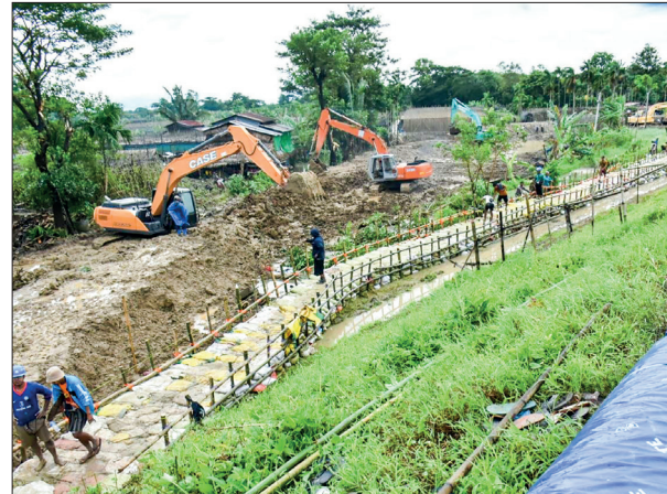
Combined forces use heavy machinery to reinforce the Nyaungdon Embankment.
