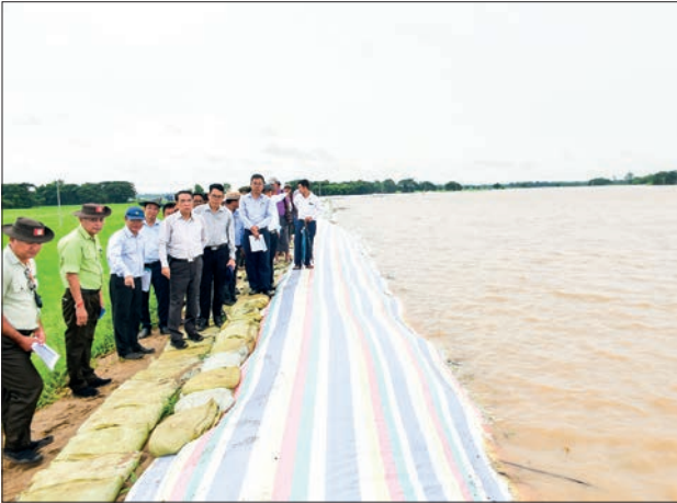
Officials inspect flood protection works and prevention of erosion along the Ayeyawady River in Letpadan Township.
