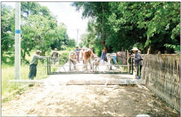
This image displays an ongoing concrete paving project in Pobbathiri Township.
