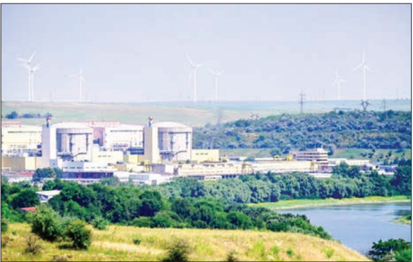
The Cernavoda plant usually generates a fifth of Romania’s electricity. PHOTO: AFP
