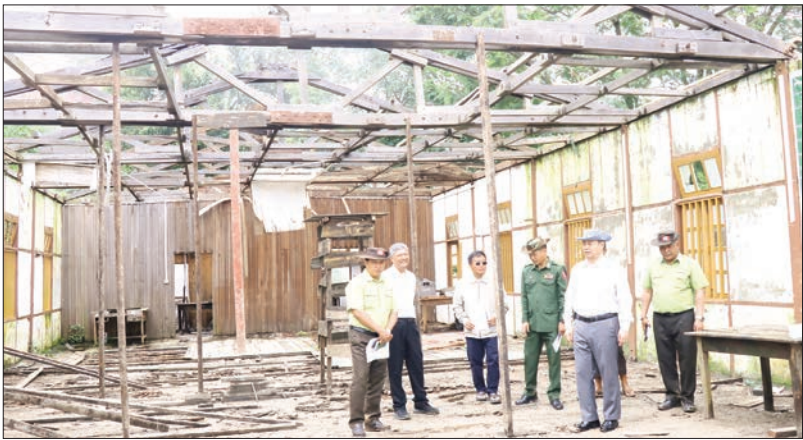
Deputy Minister Maj-Gen Kyaw Swa Oo and officials inspect the renovation work in Falam, Chin State.
