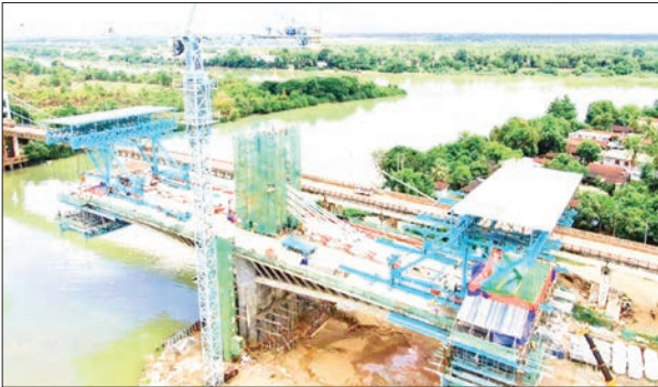
The Gyaing (Kawkareik) bridge on the Yangon-Myawady Road under construction by Japanese loans.
