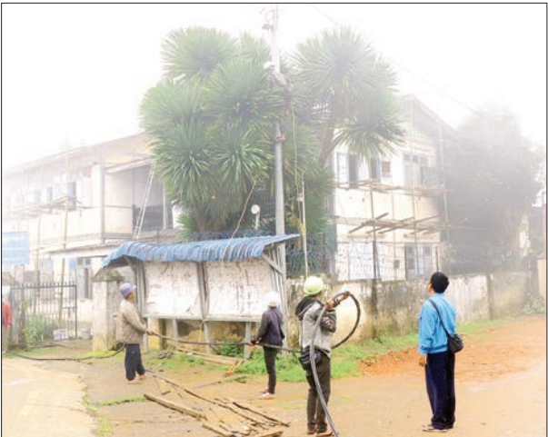
MOEE personnel are seen in the restoration of power lines.
