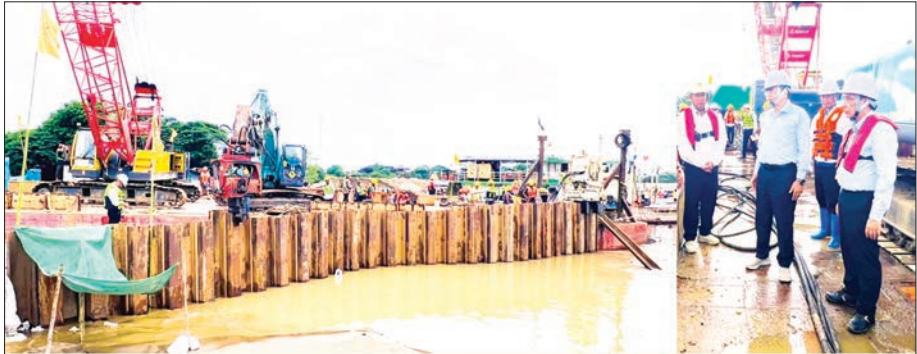
Deputy Minister Dr Thaung Naing and officials inspect the reinforcement work at the Ngawun embankment.
