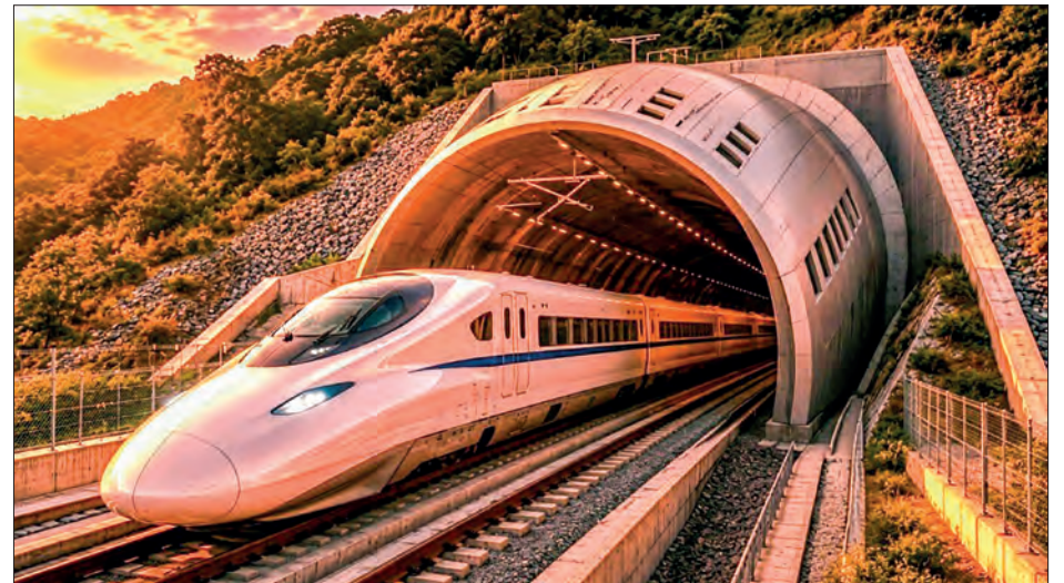
This image depicts the Mumbai-Ahmedabad high-speed rail corridor featuring advanced tunnel hood technology designed to manage air pressure and reduce noise for trains operating above 300 kilometres per hour. PHOTO: XINHUA
