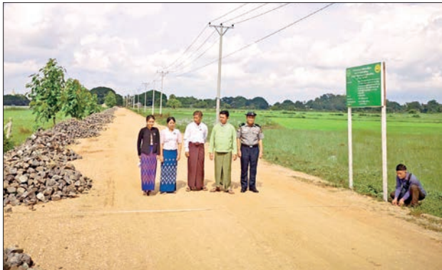
Officials are seen alongside the ongoing road construction in Kanma Township, Magway Region.
