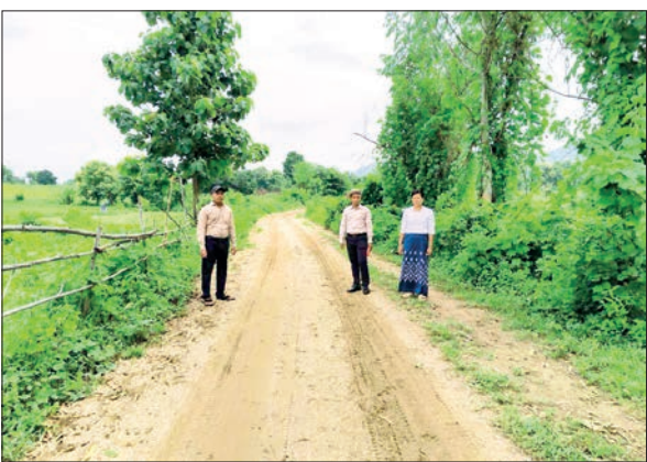
Officials are seen at a road construction project in Thayet Township.
