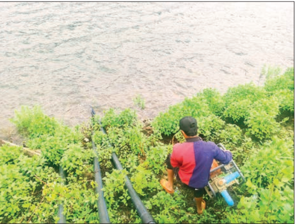
The restoration efforts of water supply are in progress in Falam, Chin State.
