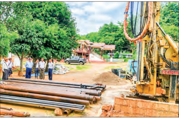
Officials from the Department of Rural Development are seen tube-well drilling in Taunggyi Township.
