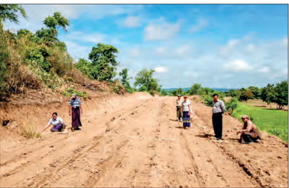
Officials from the Department of Rural Development inspect the progress of a rural production road in Aunglan yesterday.
