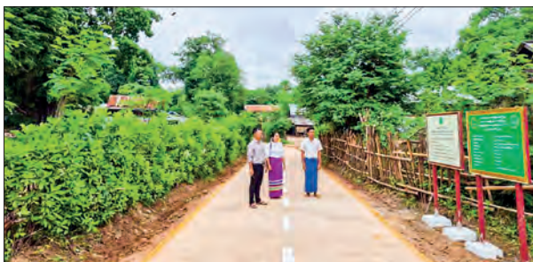
Officials from the Department of Rural Development inspect the completion of a concrete road in Kyaukpadaung Township.
