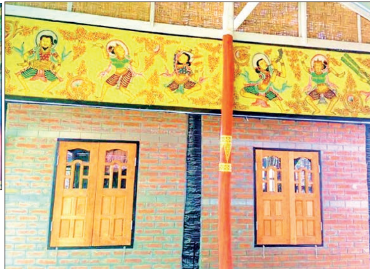
Bagan hospitality businesses display historic interior mural paintings to preserve local heritage. PHOTOS: ZWE MARN
